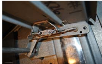
Above. Fusible link and attachment arm detail.
