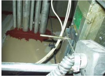
Actuator removed exposing mounting plate and damper shaft.
