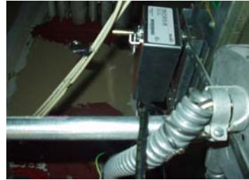
Belimo FSLF direct coupled to shaft.
