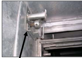
Negator spring holder. (Spring missing.) Replace it or damper.
