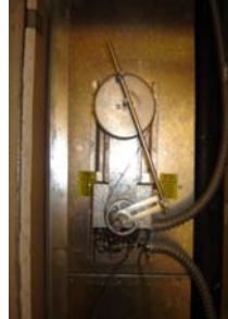
Motor with external springs
