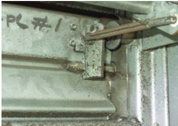
Fusible rod melts at 165°F.
