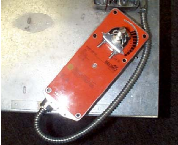
Finished mounting and wiring.
